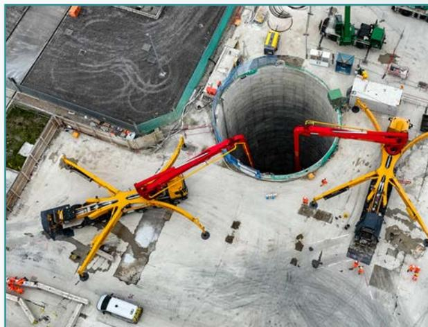
On April 22nd (Earth Day) the London Power Tunnels project saw the largest ever continuous pour of Earth Friendly Concrete®. The cement-free concrete was used to fill the base of the 55m deep tunnel drive shaft at National Grid's Hurst Substation. Its use had been driven forward by a team of young engineers and supported by contractor HOCHTIEF-MURPHY Joint Venture (HMJV). It's just one of the measures being taken by National Grid to reduce the environmental impact of construction.
